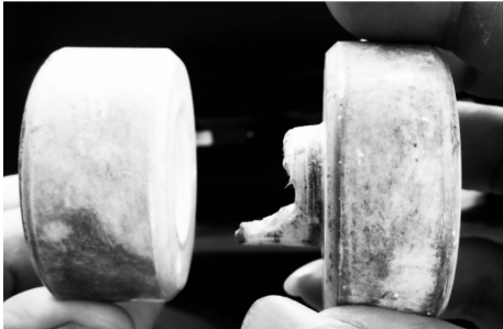
图 2 1984 号避雷器绝缘底座破损、积污情况 Fig. 2 No. 1984 insulation base damaged and polluted conditions
